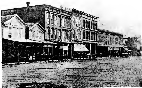
EAST SIDE COURT HOUSE SQUARE, 1869, BRYAN
